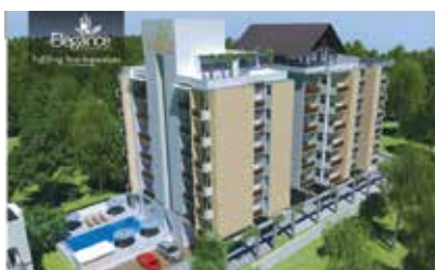
Green Elegance Thalawathugoda No of units - 54 Completed
