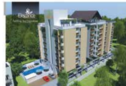
Green Elegance Thalawathugoda No of units - 54 Completed
