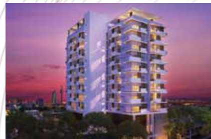
Aurum Skyline Residencies Jawatta No of units - 45 Completed
