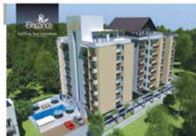
Green Elegance Thalawathugoda No of units - 54 Completed
