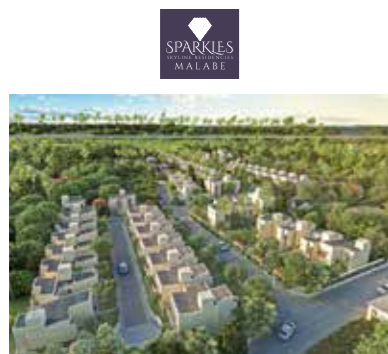
Sparkles Skyline Residencies - Malabe No of units - 83 Completed
