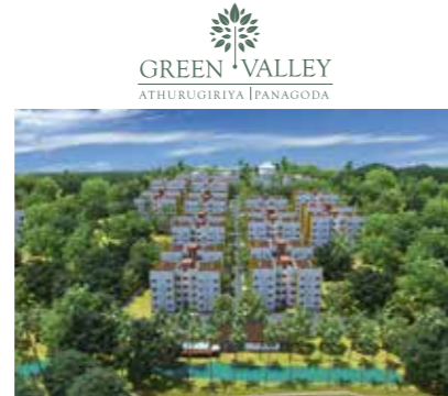
Green Valley Athurugiriya Panagoda No of units - 354 Completed
